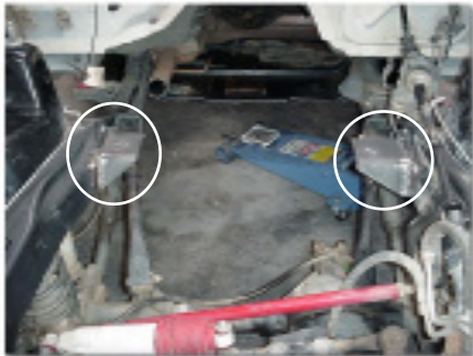
New frame mounts welded into position
