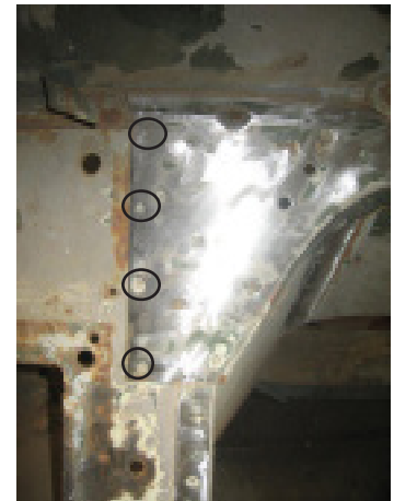
Bulkhead spot welds
